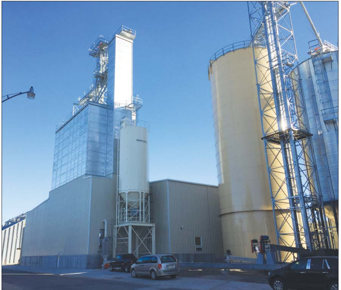
Farmers Ranchers Co-op Association's new feed mill in Ainsworth, NE, the second of two on the South Main Street site. Photo courtesy of EBM Construction Inc.
