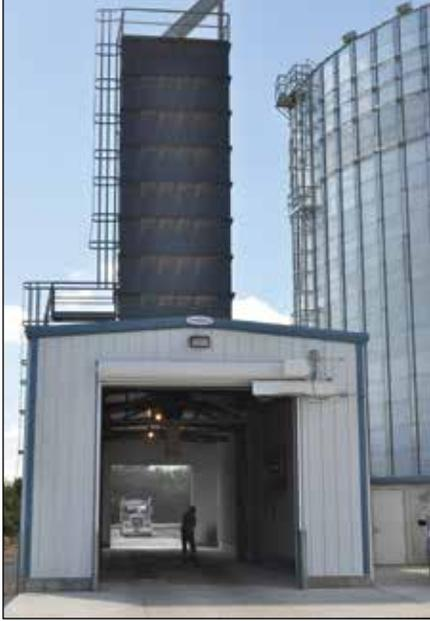
*New receiving pit features a dump-through truck scale that reaches a 20,000-bph receiving leg.*
