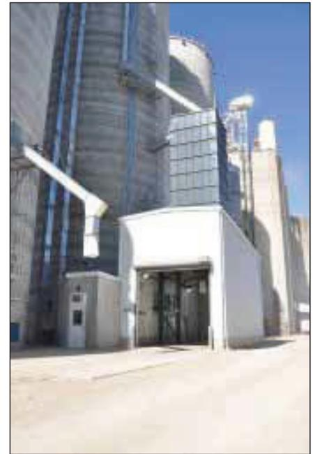
tanks have additional 30-hp fans and one a 50-hp fan for air-assisted unloading. The project also includes a 1,000-bushel enclosed mechanical receiving pit, one of three at Hinton. It feeds grain into a 20,000-bph Schlagel receiving leg equipped with a single row ►
