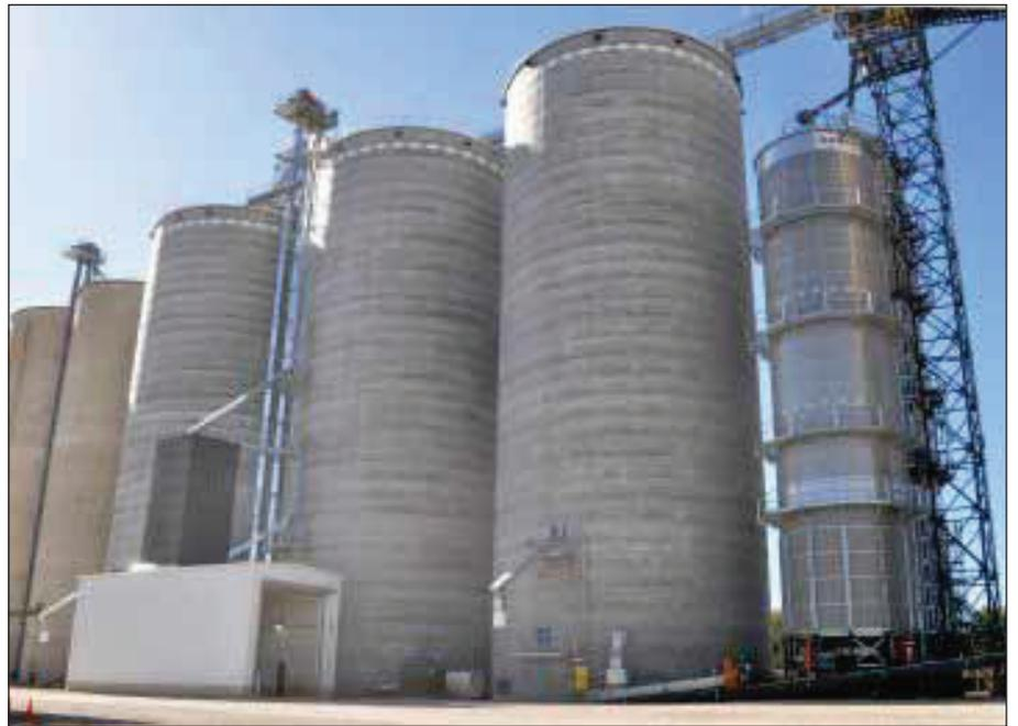
*Closeup view of three new McPherson jumpform concrete tanks, receiving pit, and Schlagel leg, and a Brock 4,700-bph tower dryer (not pictured is a Brock 4,000-bph dryer). Ground-level photos by Ed Zdrojewski.*
