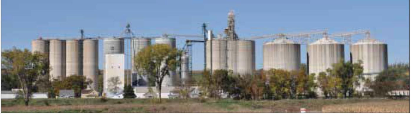
*Central Valley Ag's rail terminal at Hinton, IA, above, with three new McPherson jumpform concrete tanks and a Schlager receiving leg visible just left of center. Below right, an AIRLANCO centrifugal fan provides power for a KanalSystem aeration and air-assist unloading floor.*
