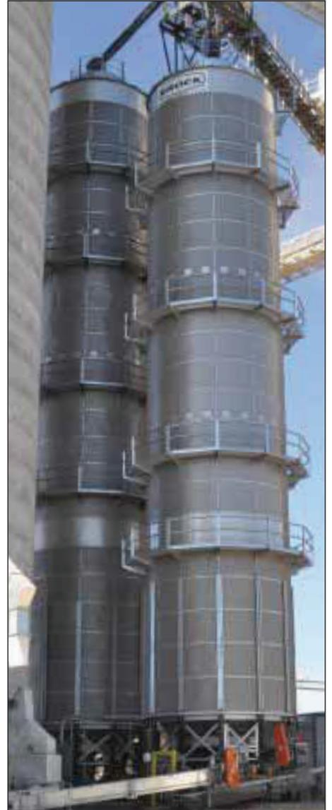
*Pair of Brock tower dryers provide 8,700 bph of drying capacity at five points of moisture removal.*
