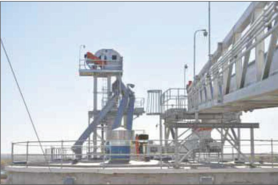
*Rooftop equipment, above, includes the head section of a Schlagel 20,000-bph receiving leg and four-hole Schlagel distributor, as well as a 20,000-bph Schlagel drag fill conveyor. At right, a new 1,000-bushel enclosed receiving pit feeds grain into the receiving leg.*
