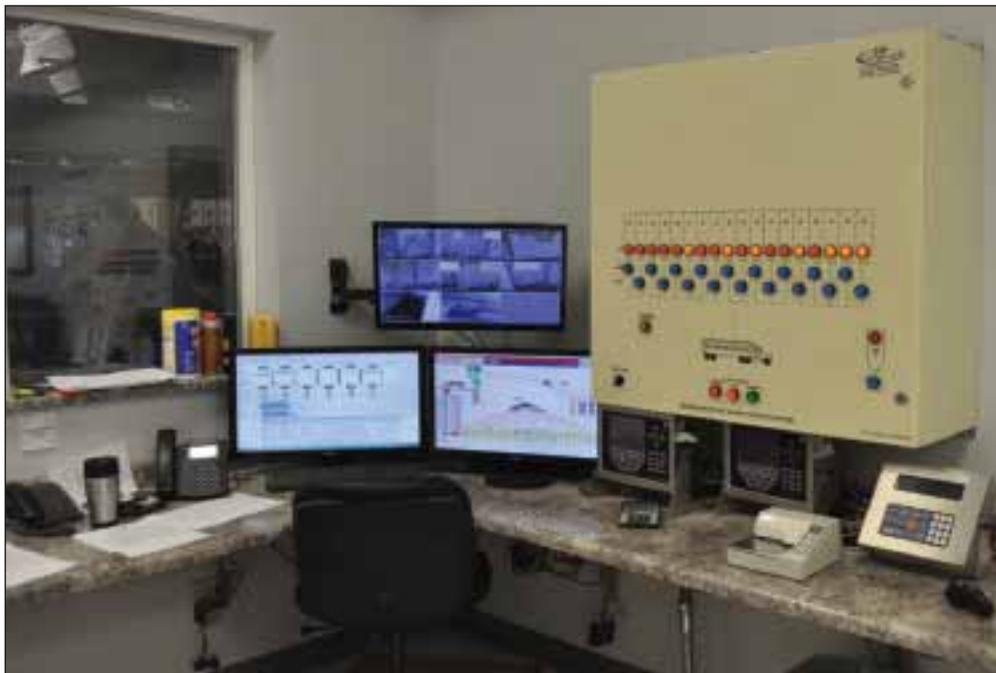
*Control room features an Easy Automation batching system, which also is used to run a new grain elevator next door.*
