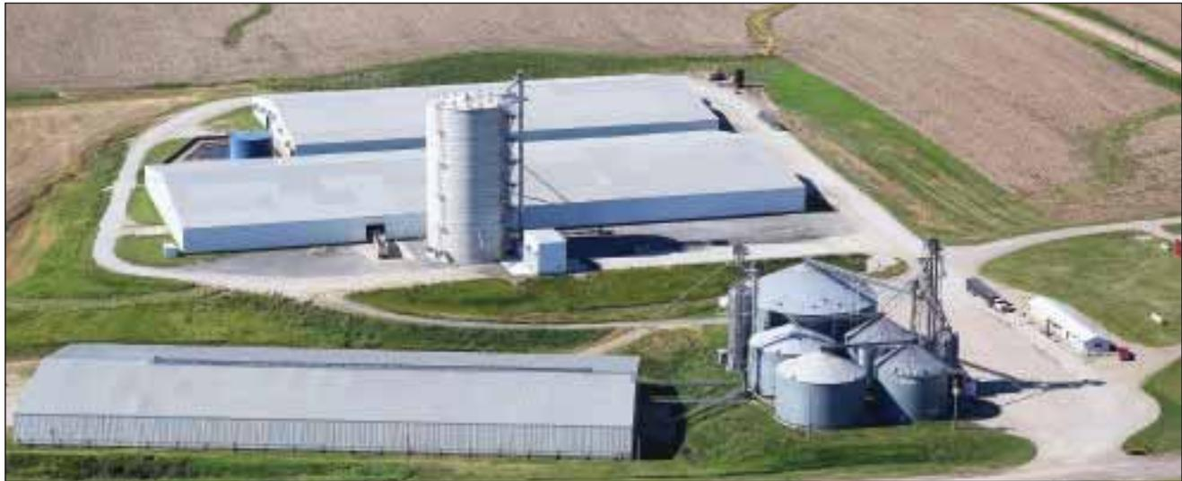
*Cooperative Supply Inc.'s grain elevator at Dodge, NE, with new jumpform concrete storage silo and freestanding leg adjacent to a 2-million-bushel soybean flat storage. Aerial photo courtesy of Dakota Aerials, Yankton, SD.*
