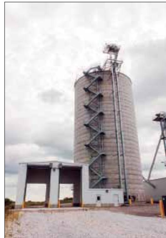
*Ground-level view of the new annex with twin enclosed receiving pits, Hoffmann 350,000-bushel concrete storage silo with Warrior switchback staircase, and free-standing Schlagel 20,000-bph leg.*
