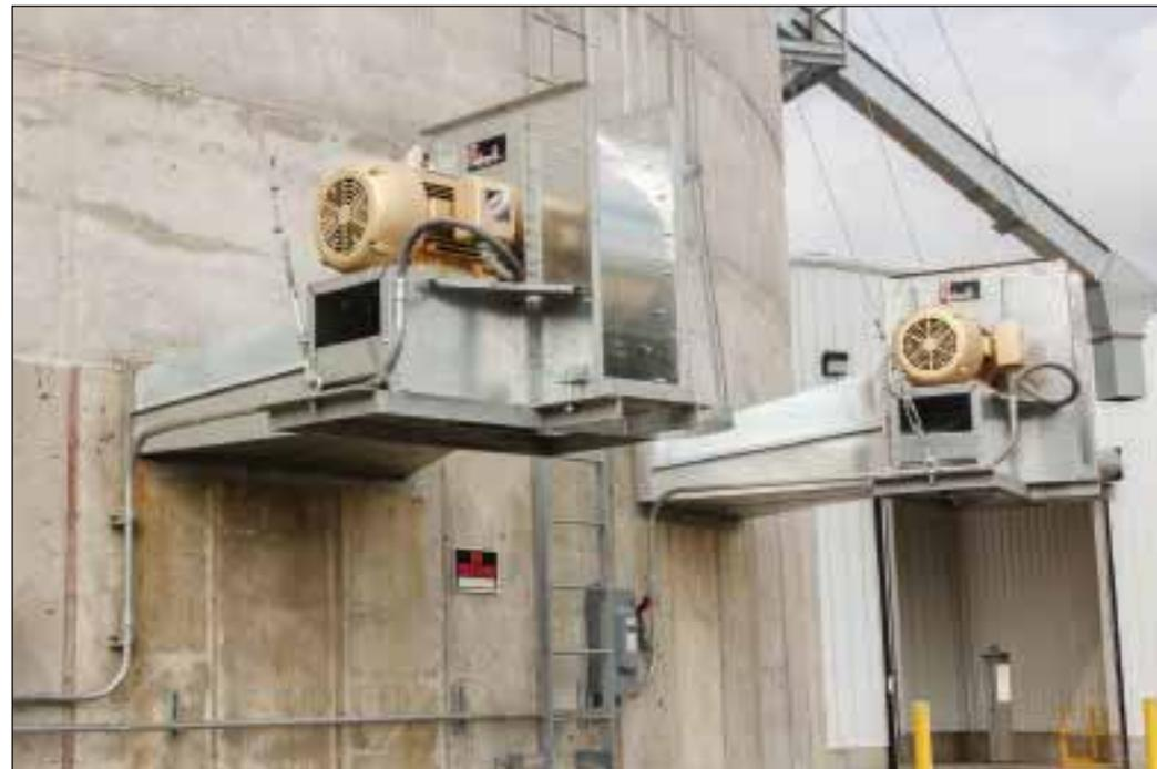
*Two of four Caldwell 40-hp centrifugal aeration fans that deliver roughly 1/10 cfm per bushel to stored grain. Ground picture courtesy of EBM Construction.*
