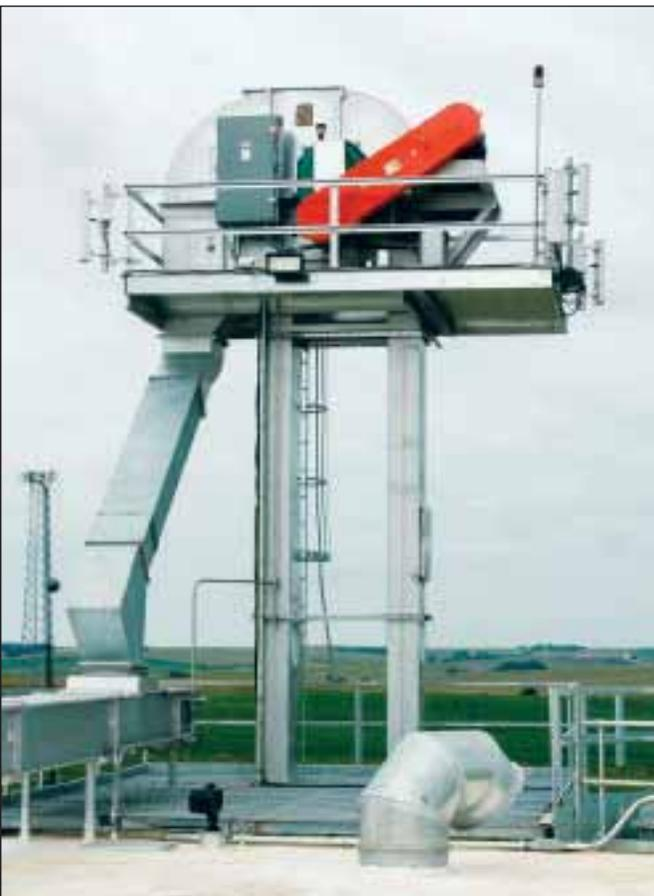
*Head section of the new 20,000-bph Schlagel receiving leg from which grain can go to the new concrete storage silo.*
